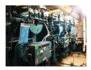
GS-04P-11-EX-C-0064 Design/Build Services For Boiler Replacement - Freeland completely removed the existing boilers and replaced them with high efficiency boilers. While the building was built around the original boilers, Freeland designed and implemented a solution that required no modifications to the exterior of the facility. This work was completed with no impact to courthouse operations (Savannah, GA GSA)
