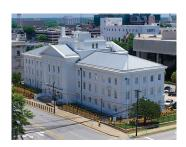
GS-04P-12-EX-00070 - Freeland is providing Design/Build Services for the complete exterior renovation of 1930's era Bankruptcy Courthouse. This work included remediating the asbestos in the window frames, painting the exterior, retrofitting the gutter system, replacing the built up roof in its entirety, and providing new landscaping. (Columbia, SC GSA)
