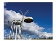
FA4418-12-P-0106 Demolition of Water Tower at ASLAC – This project was performed in the middle of an existing Army Ordinance Area at the Naval Weapons Station. Due to the geometry and weight of the lifts, a 400 Ton Hydraulic Truck Crane with a Luffing Jib was utilized to perform this job in a efficient and safe manner. (USAF - Joint Base Charleston)
